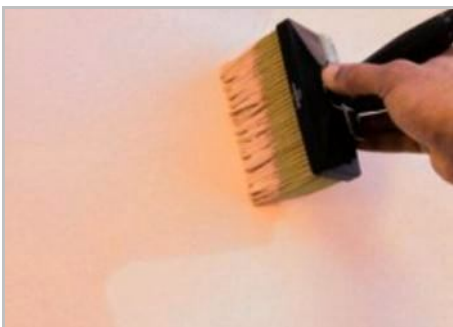
Step 5 - Second coat by "pull and blend"
