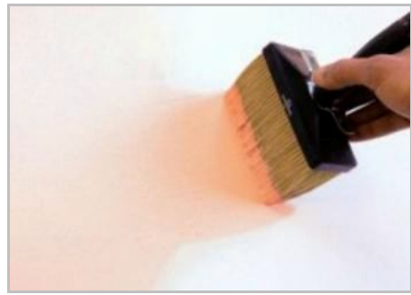
Step 4 - First coat by "pull and blend"
