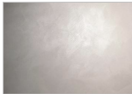
Step 6 - Let the product dry. A second coat would make the effect more opaque and homogeneous
