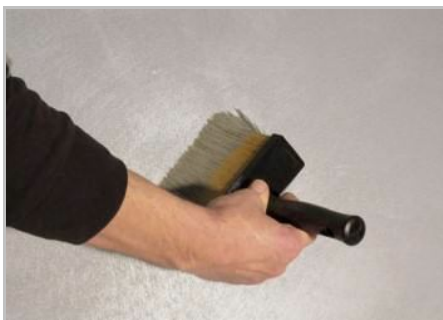
Step 5 - After several minutes, caress the product with a dry brush if you want to uniform the drawing
