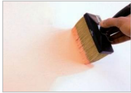
Step 4 - First coat by "pull and blend"
