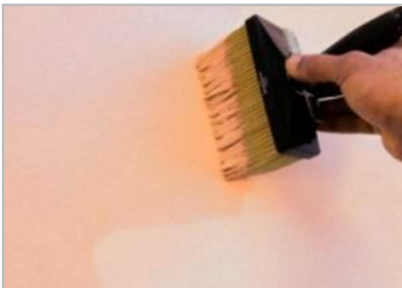
Step 5 - Second coat by "pull and blend"
