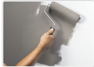
Step 3 - Apply the first coat with a roller (PE15), coverage 8/10 m 2 /lt each coat
