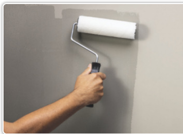
Step 5 - After at least 12 hours, apply with a roller (PE15) Vetro Opaco diluted 30% with water. Coverage 15/18 m 2 /lt
